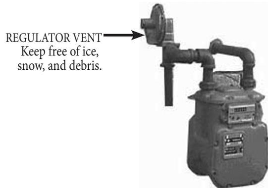
It is important for these vents to remain clear. Do not allow moisture, which could freeze, to build up in the vent. If you see moisture building up in the regulator vent, contact your gas supplier.
