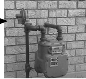
Figure 1 - Gas Regulator Vent
