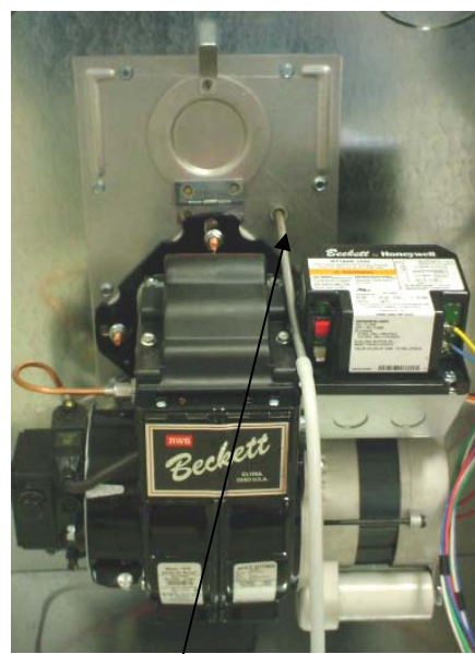
Over-fire draft access port.
