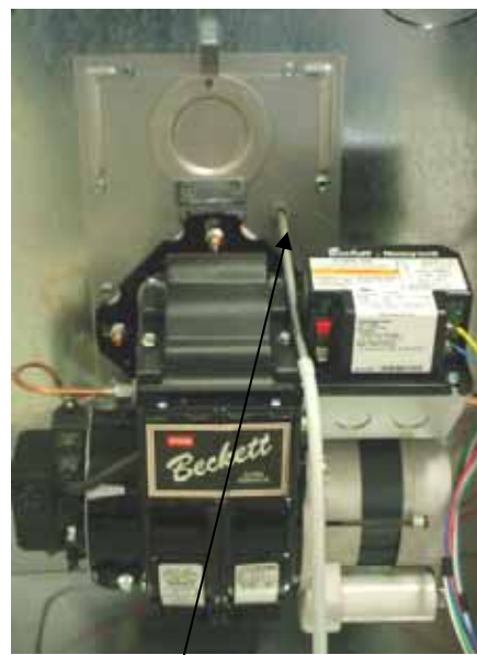
Over-fire draft access port.
