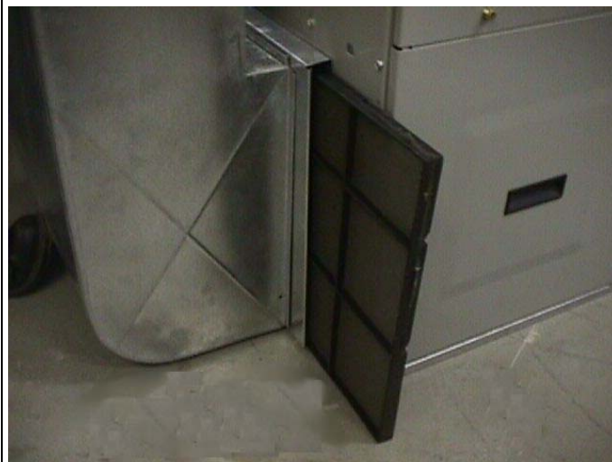
Figure 22: Air filter Maintenance.
