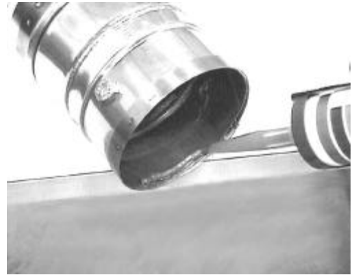
Applying bead of silicone to the female portion of the appliance / vent adaptor.
