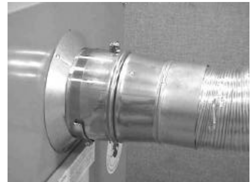
Typical Appliance Connector with test port.
